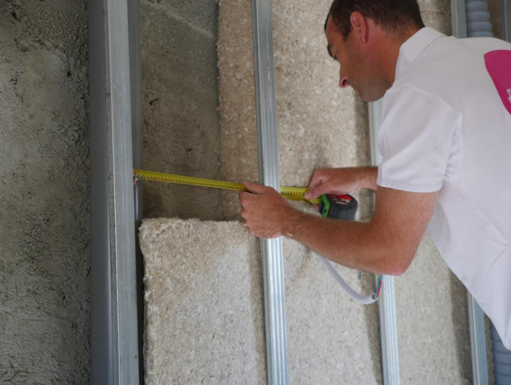
Pose isolation @Biofib
